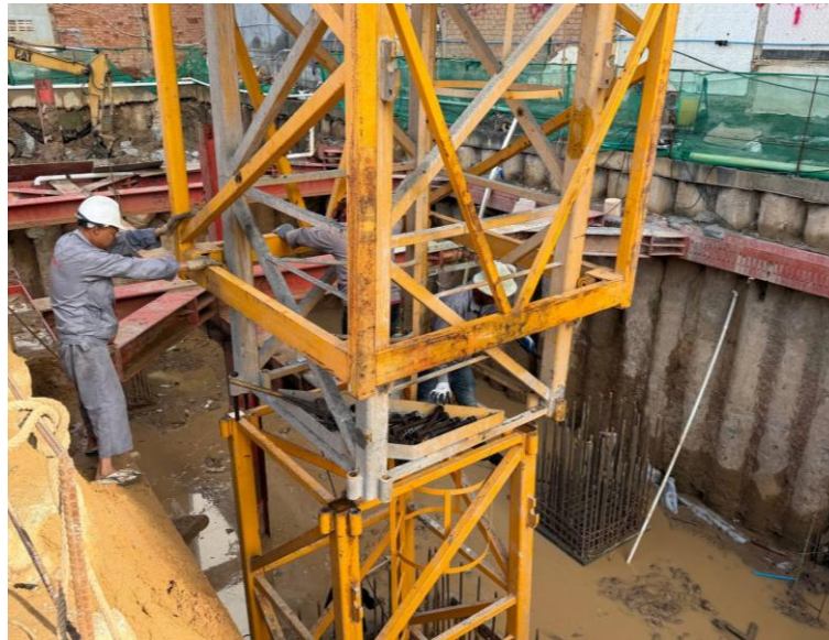
Tower Crane Installation
