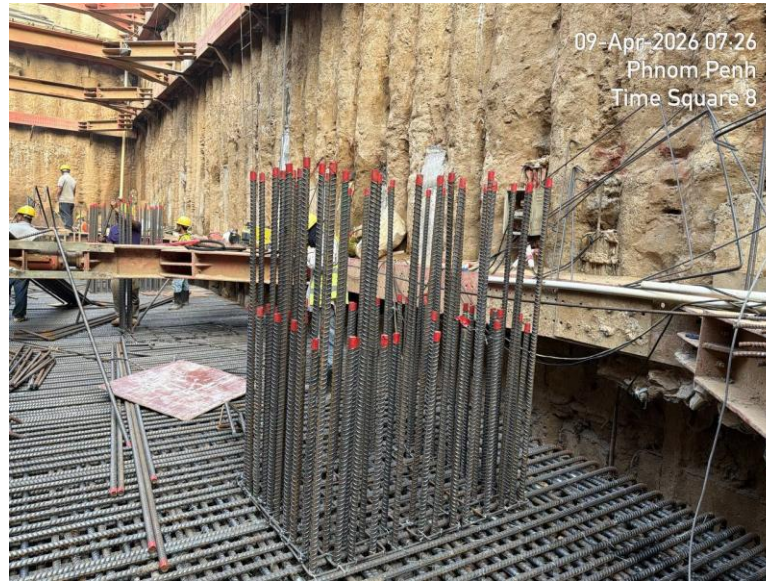
Inspection of Columns Starter Bars & Boundary
