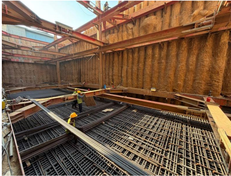
Inspection of Top & Vertical Bar
